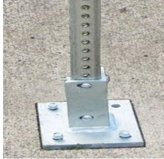
Figure #45: Sign being mounted into the concrete
